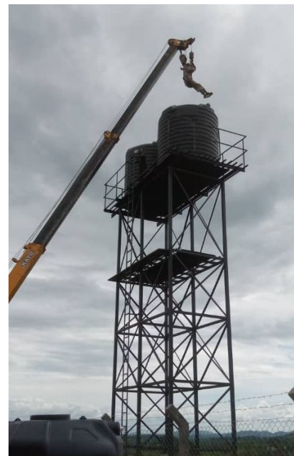
The elevated water tanks just installed at the high school carry water by gravity throughout the campus and to a tap for the community to access our harvested water when we have enough to share.
