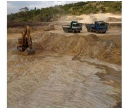
The reservoir is massive taking 45 days of heavy machinery work to create.
